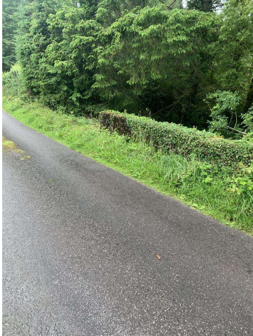
General view of the east parapet
