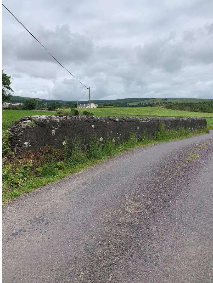
General view of the bridge parapet
