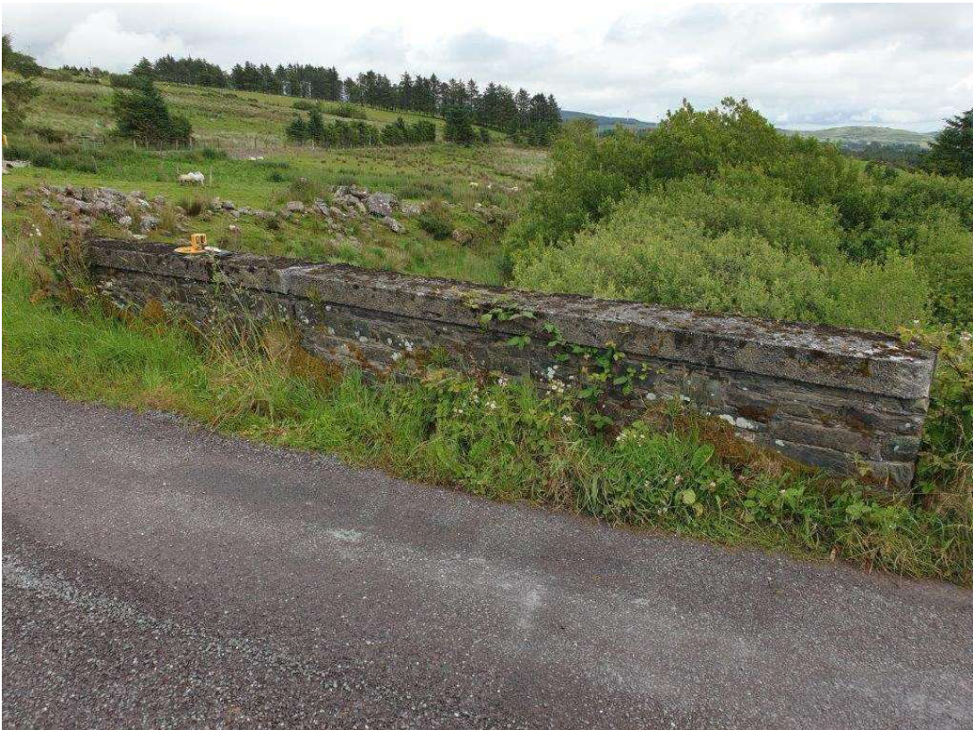
General view of the east parapet
