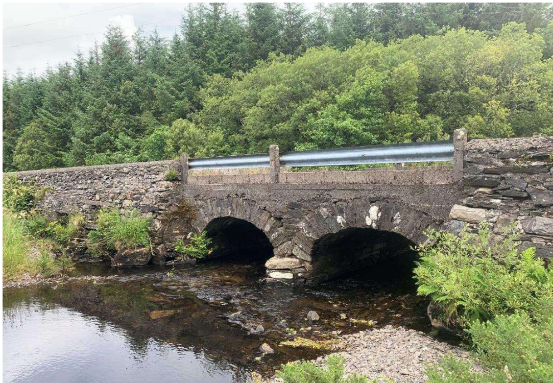
General view of bridge elevation
