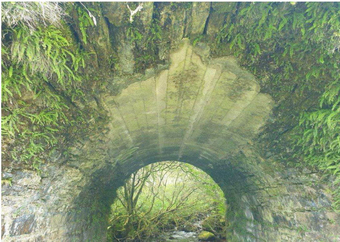
General view of the arch barrel from the east
