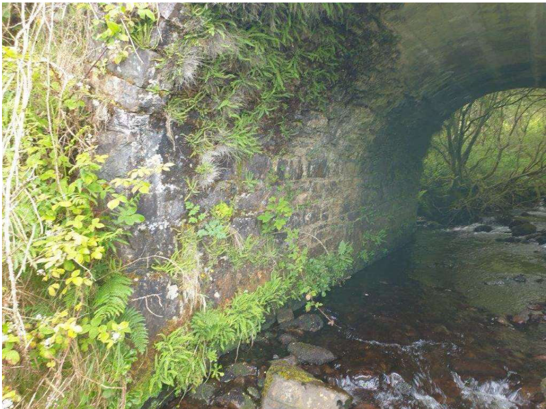
General view of the south abutment
