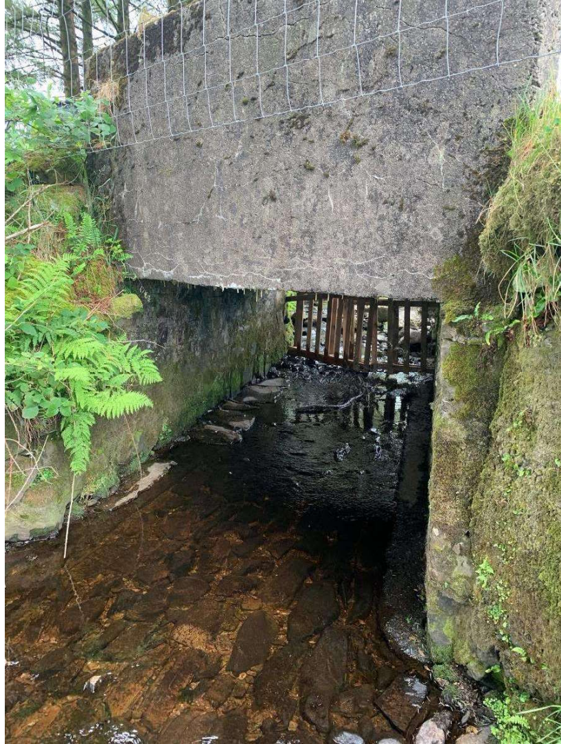
General view of the bridge elevation
