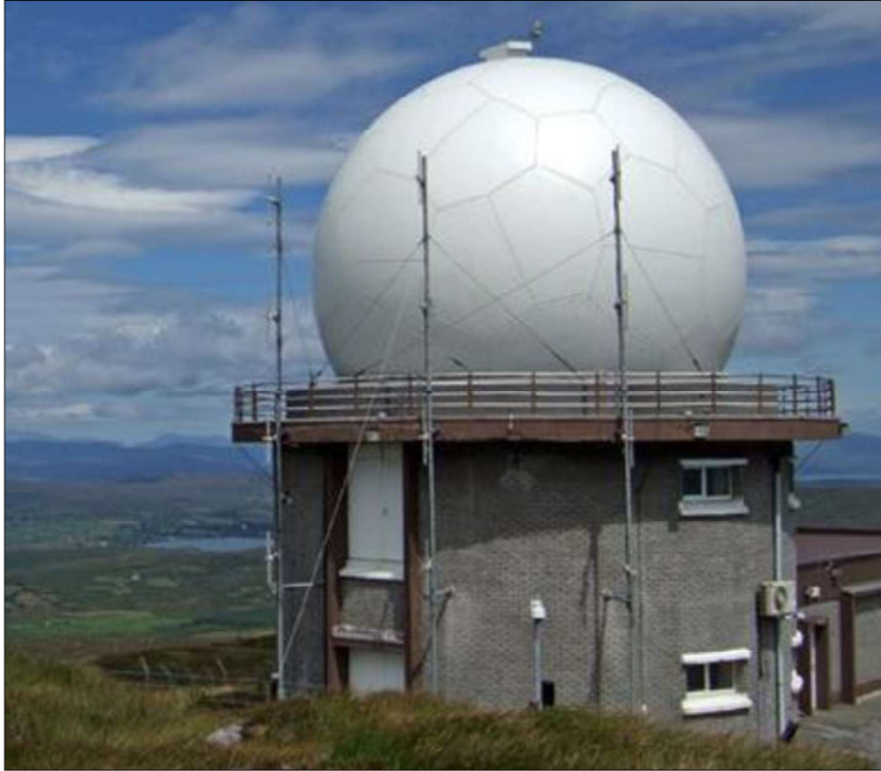
Figure 9. Mt Gabriel Radar Station.
