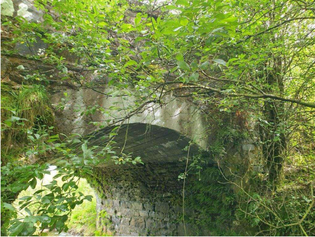
General view of the west elevation
