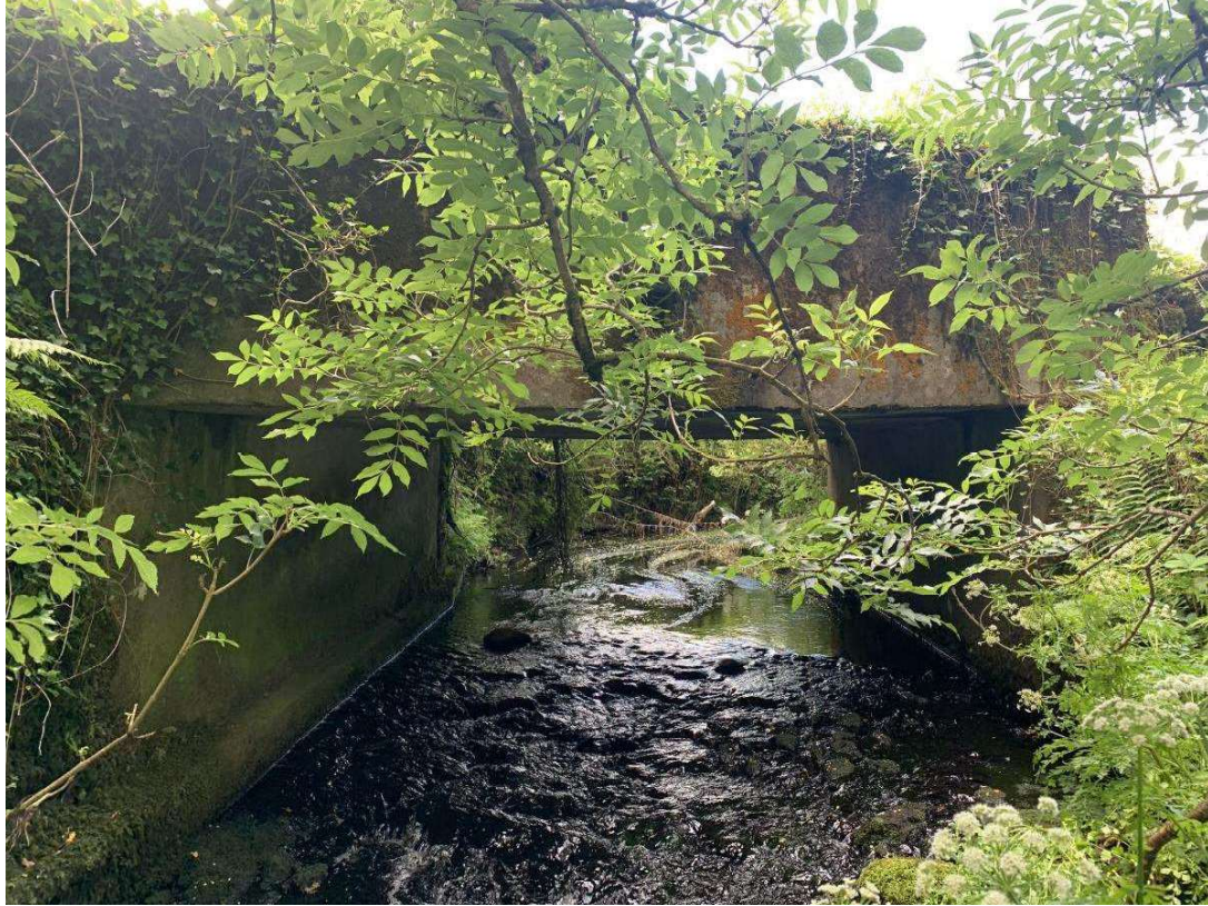
General view of the bridge elevation
