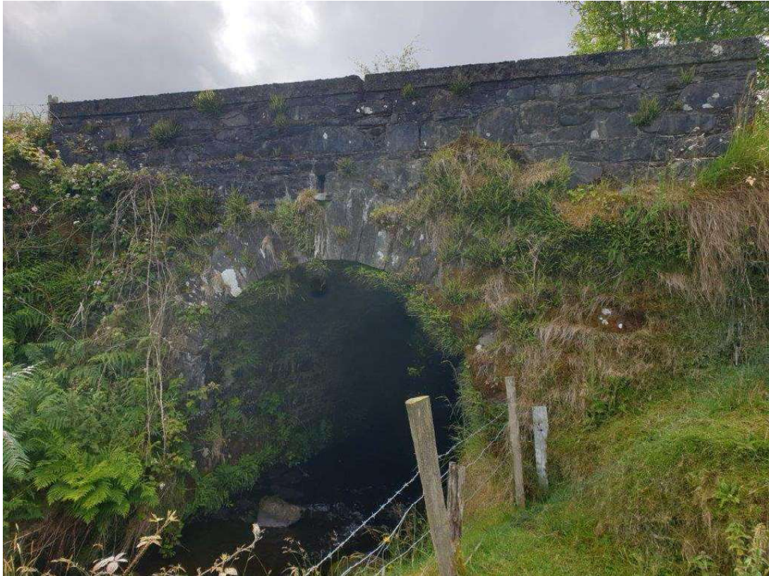
General view of the east elevation
