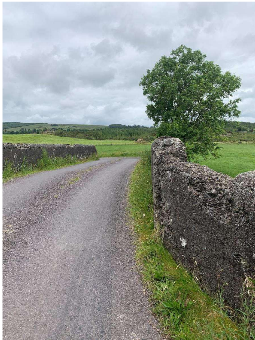
General view of the bridge surface
