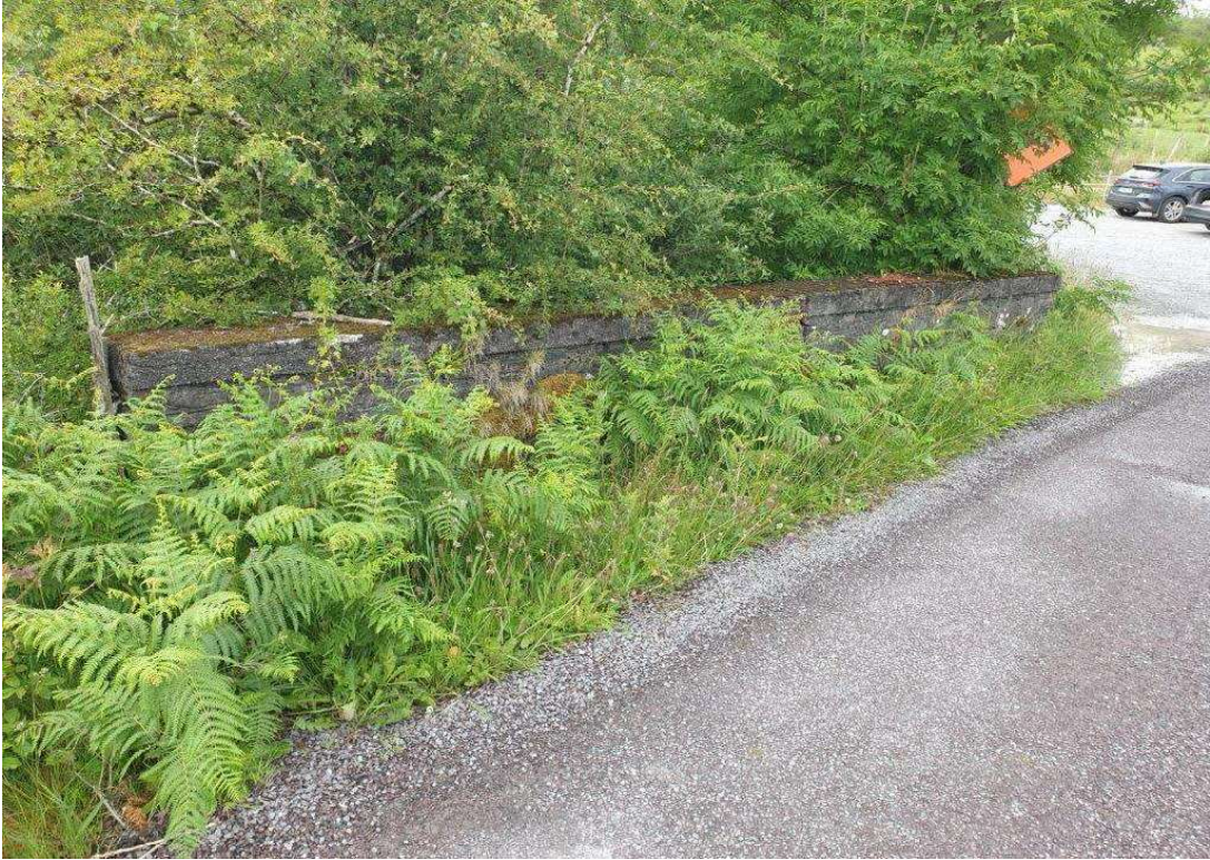
General view of the west parapet
