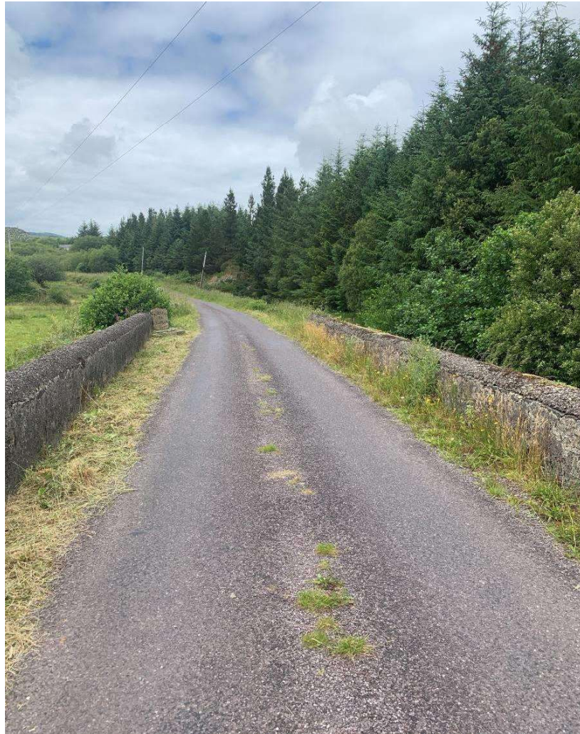
General view of the bridge surface
